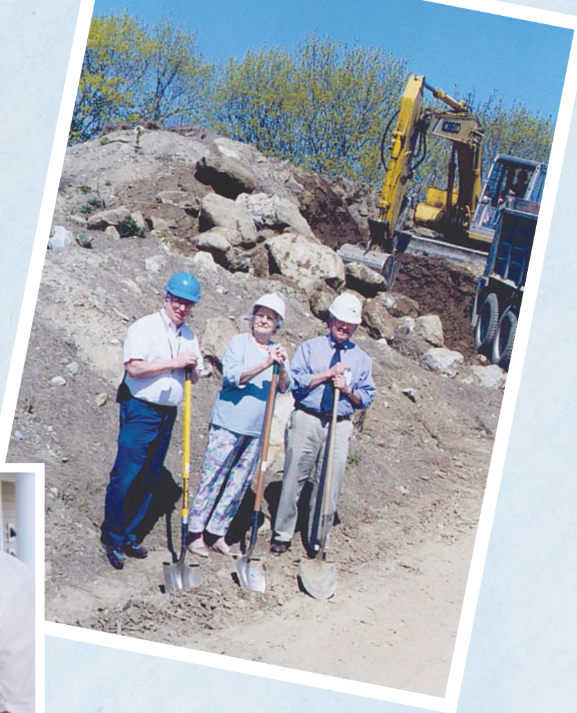
Bob Nault (left), a future resident, and Bob McKeown appear ready to join excavators in the construction zone. Quarry Hill's first physical plant director, Nault stepped out of retirement to oversee development of the $30 million project.
